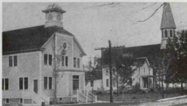
ST. MARY'S R. C. CHURCH Erected during 1886
