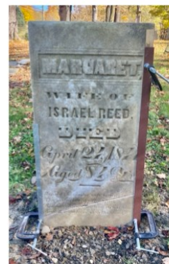
The tablet is "welded" back together using historical stone epoxy, then braced for stability while it cures.
