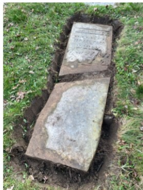
The full length white marble tablet of Margaret Reed after a trench was dug around stone for cleaning and to assess proper repair strategy.
