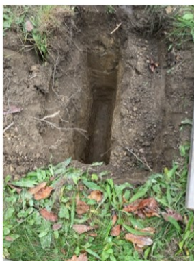
A 30" deep x 8" wide trench was dug to set the bottom 40% of the tablet. Gravel was added to the bottom to prevent the marble from sitting directly on the clay ground.
