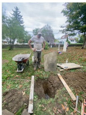
Preparing to set the bottom portion of Margaret Reed's stone in the hole. 2" of gravel lined the bottom. Brian Daddis
